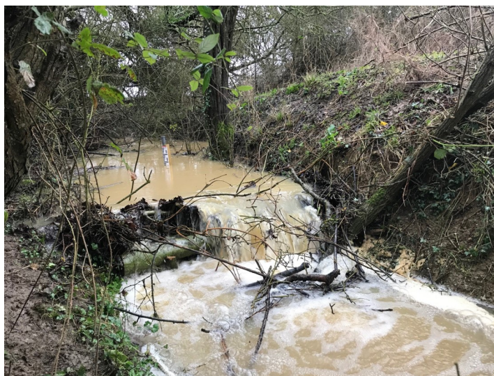
Figure 3. Fixed large wood in-channel leaky barrier storing water during high flow event (© Dave Gasca-Tucker)
