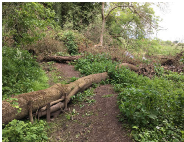
Figure 1. An example of a basic overland leaky barrier on the River Soar NFM Pilot Scheme, made from a single tree trunk (© Atkins Ltd)
