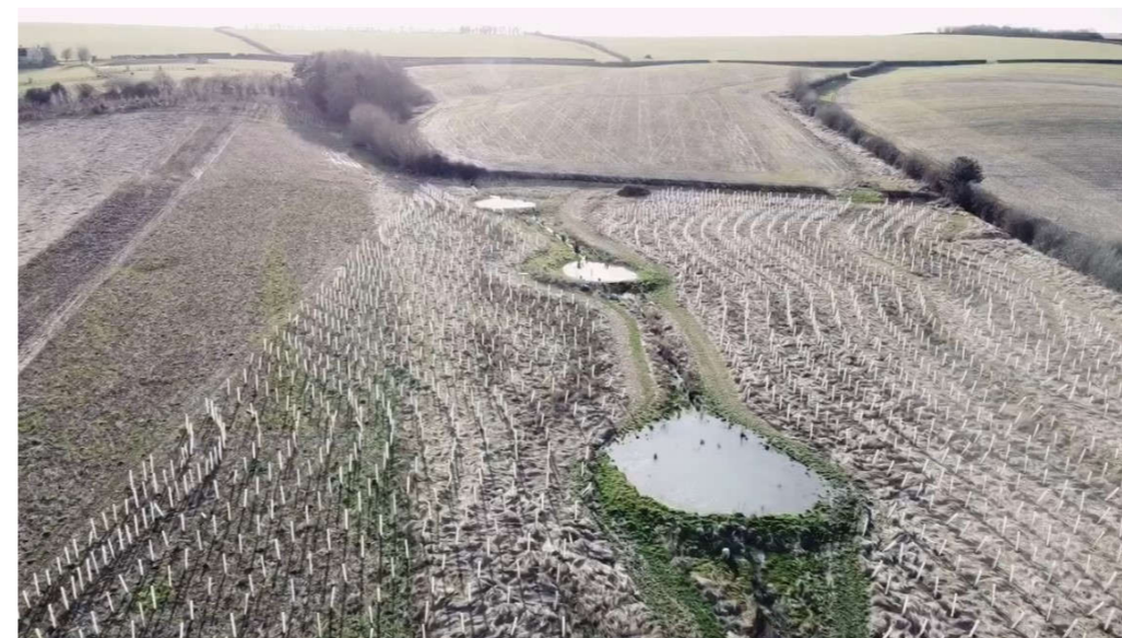
Figure 3. Online storage ponds with adjacent tree planting as part of the Evenlode NFM scheme (© Evenlode catchment Partnership)
