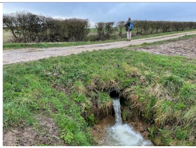
Photo 05. Piped ditch connection
