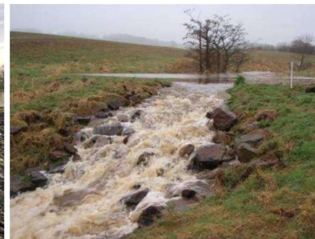
Figure 2. An online storage pond within the channel, complete with rock armour spillway (© Newcastle University)
