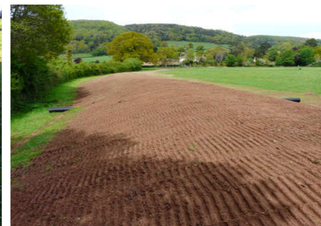
Figure 5. A cross-slope bund with outlet pipe to reduce chance of overtopping during heavy rainfall events (© National Trust)
