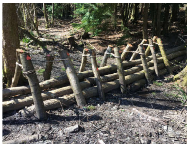
Figure 3. A multiple log overland leaky barrier, with extended in-channel leaky barrier (WC01.1) and substantial fixings (© Jay Neale)
