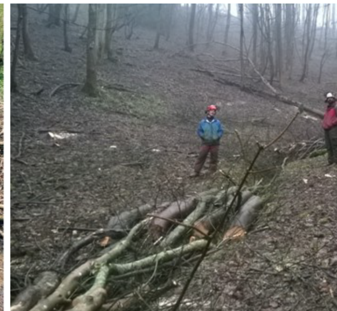
Figure 2. Headwater channel woody bundles after placement in a channel to mimic natural blockages, as part of the Stroud District Council Rural SuDS Project (© Stroud District Council)
