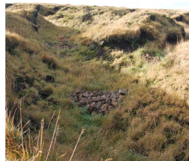
Figure 3. Stone dams blocking a gully. Vegetation has re-established within the channel following gully blockage (© Moors for the Future Partnership)
