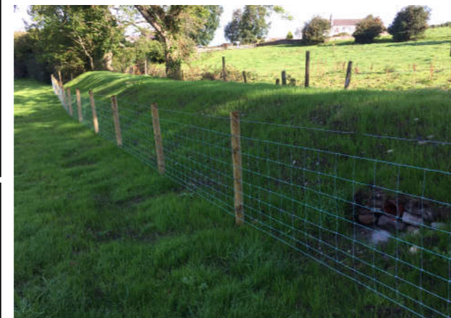
Figure 4. A cross-slope bund with fence for added protection against livestock poaching (© Cumbria County Council)
