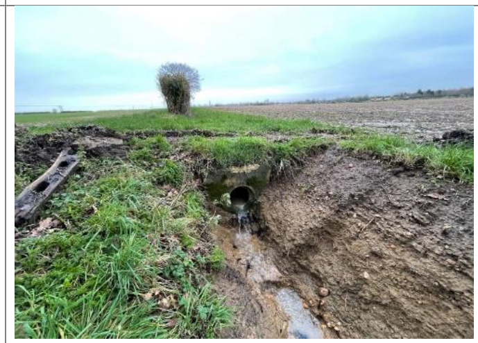
Photo 06. Piped ditch connection
