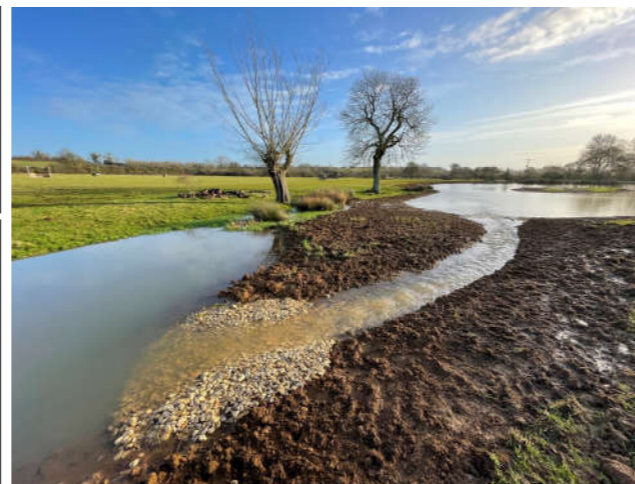
Figure 1. Online storage feature at Magpie Farm, complete with armoured spillway (© Atkins Ltd)
