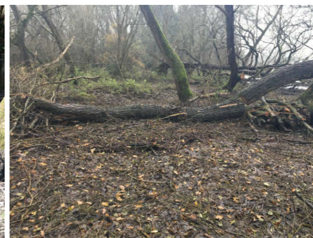
Figure 4. An example of a more complex overland leaky barrier, made from a hinged large trunk and smaller logs bundled together (© Atkins Ltd)
