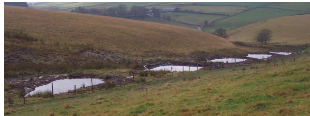
Figure 3. A series of offline storage ponds forming a wetland habitat and benefits for NFM (© Tweed Forum, Hugh Chalmers)
