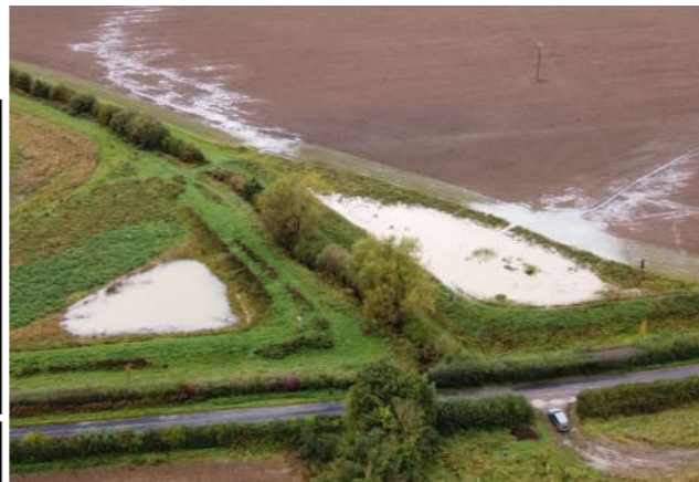
Figure 1. Flow pathway bunds strategically located to intercept overland flow before exiting fields on to a road (© Evenlode Catchment Partnership)
