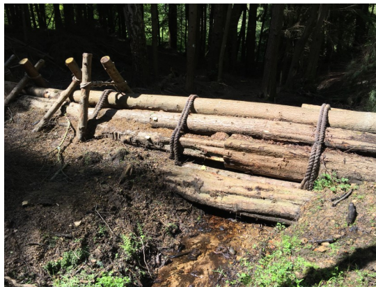
Figure 1. Formally structured in-channel leaky barrier with rope and wooden stake fixings (© Jay Neale)
