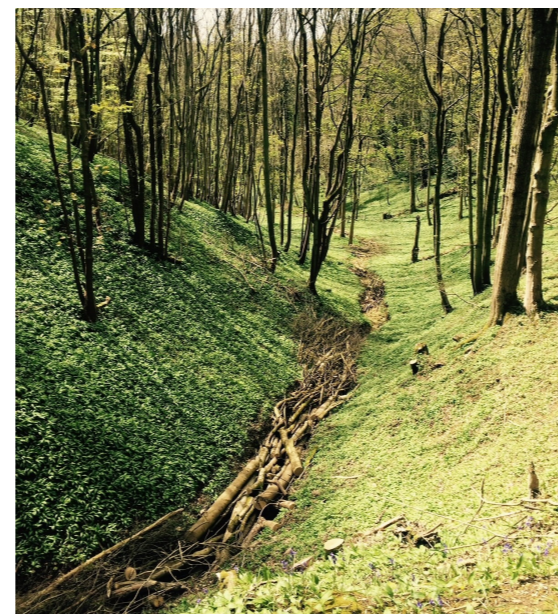
Figure 3. Headwater channel woody bundles in a wooded valley (© Dave Gasca-Tucker)
