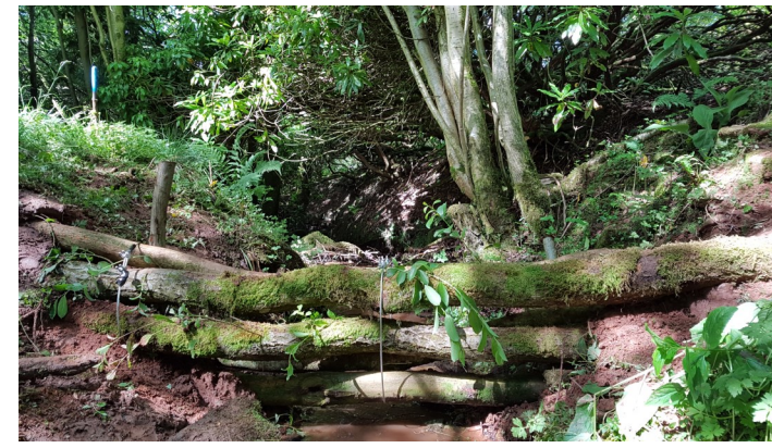
Figure 2. Formally structured in-channel leaky barrier with wire fixings and trenched into banks (© Eden Rivers Trust)
